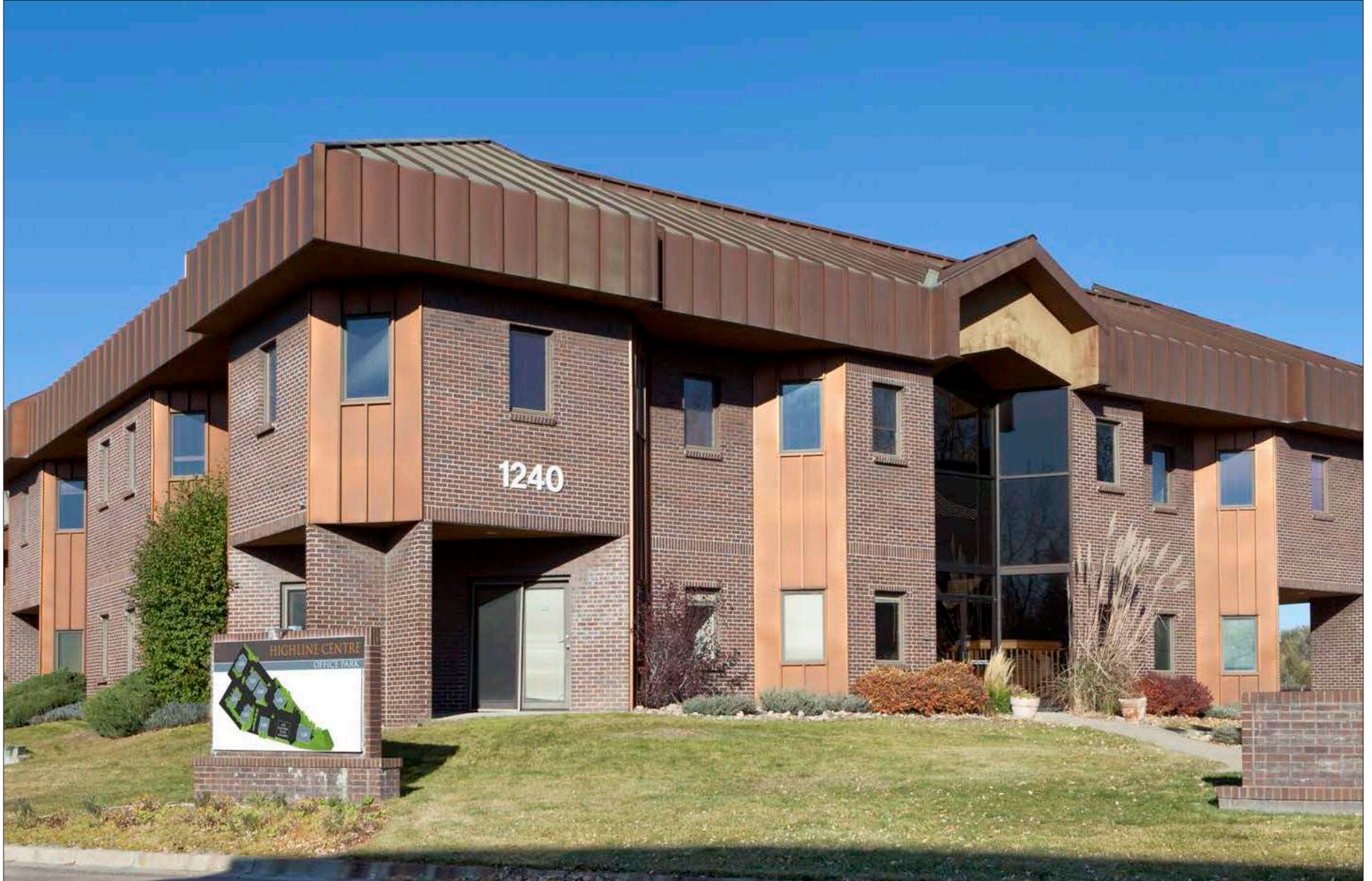
BUILDING 1240 EXTERIOR PHOTO
