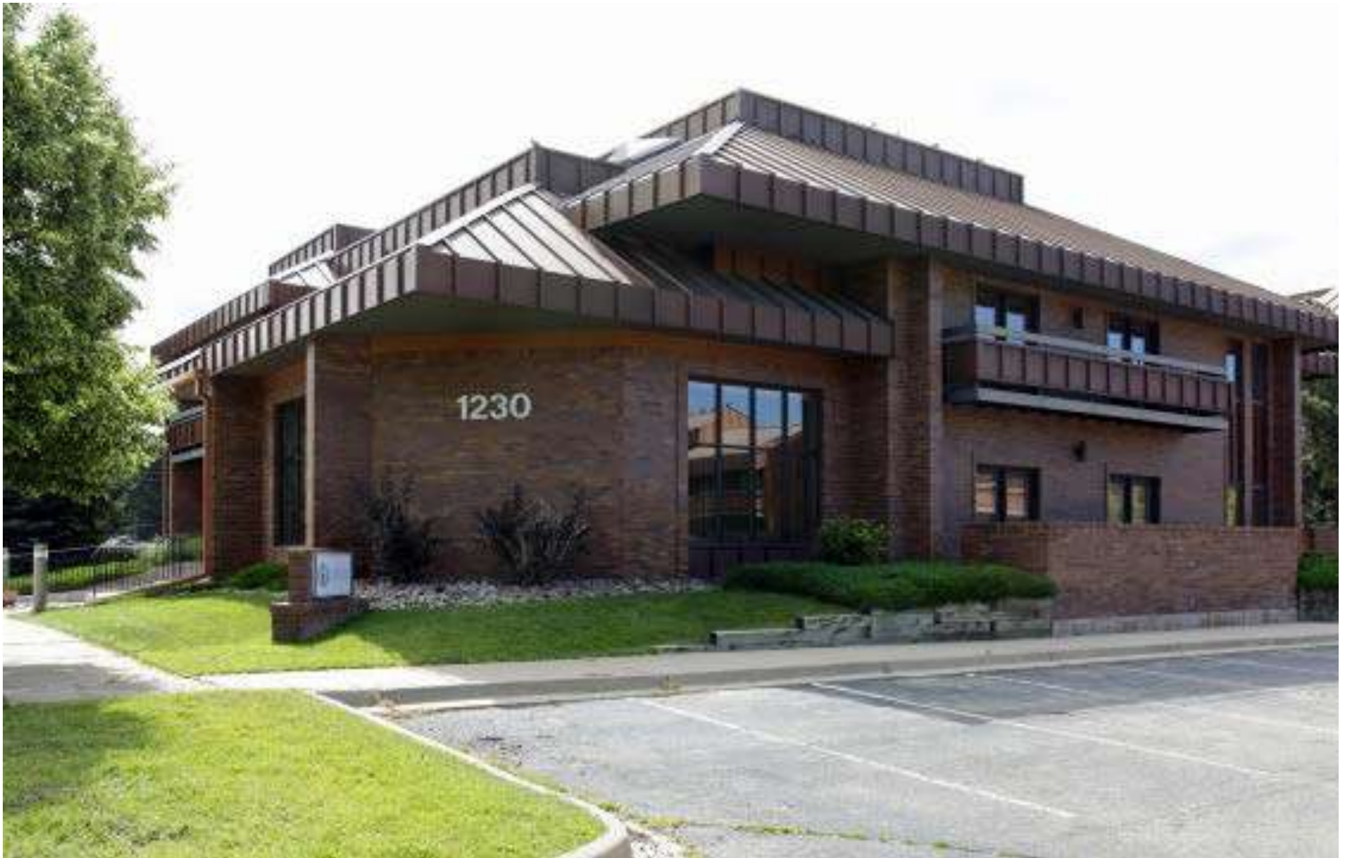
BUILDING 1230 EXTERIOR PHOTO
