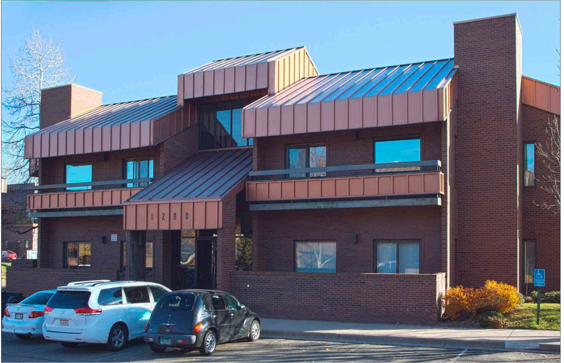
BUILDING 1200 EXTERIOR PHOTO
