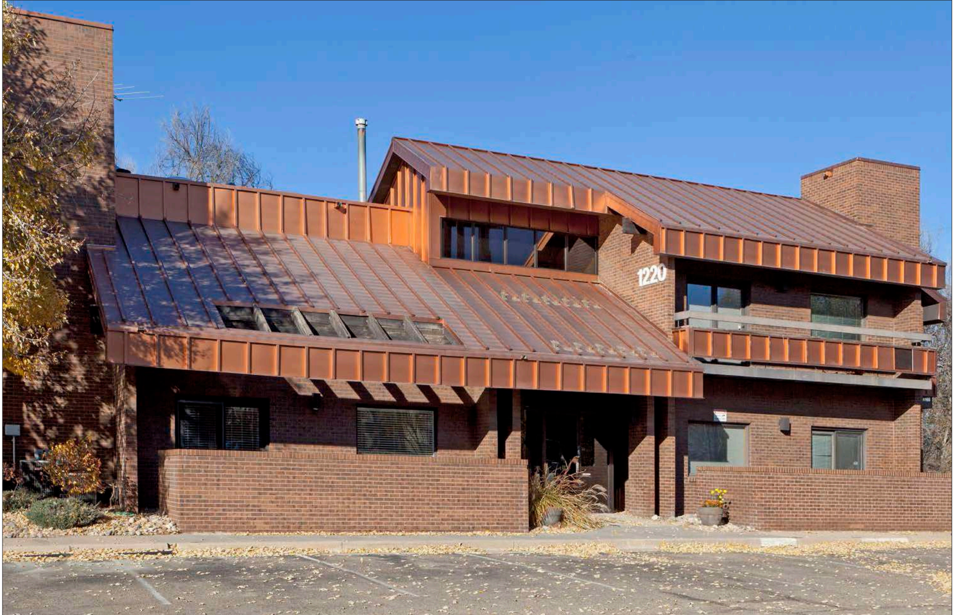
BUILDING 1220 EXTERIOR PHOTO
