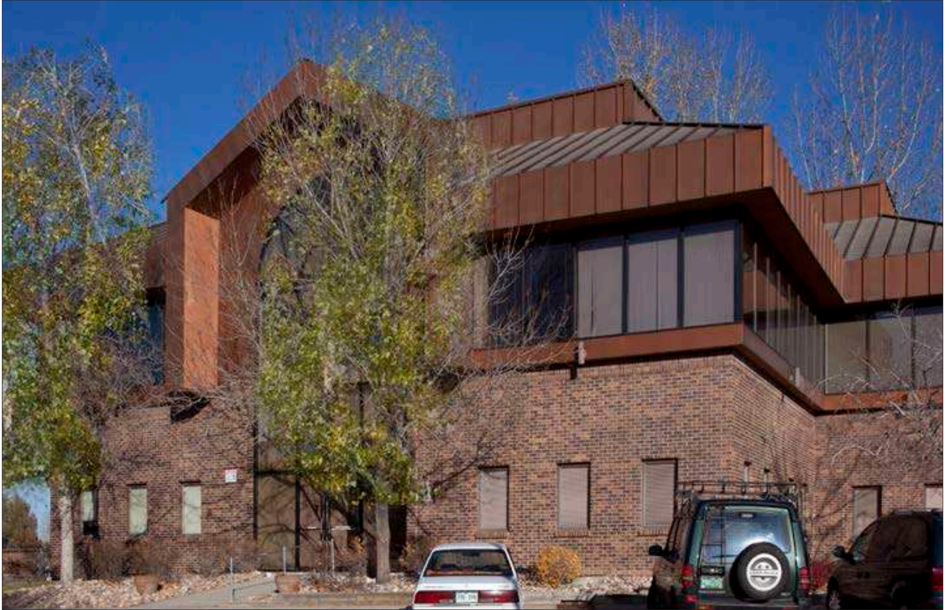
BUILDING 1250 EXTERIOR PHOTO
