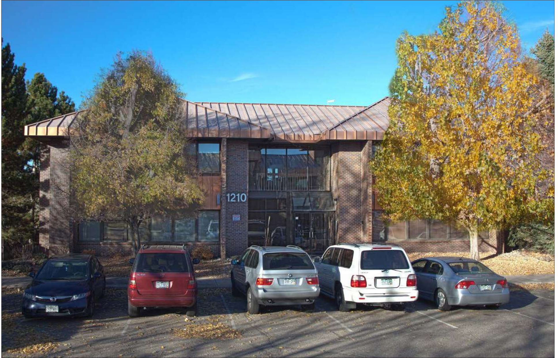
BUILDING 1210 EXTERIOR PHOTO
